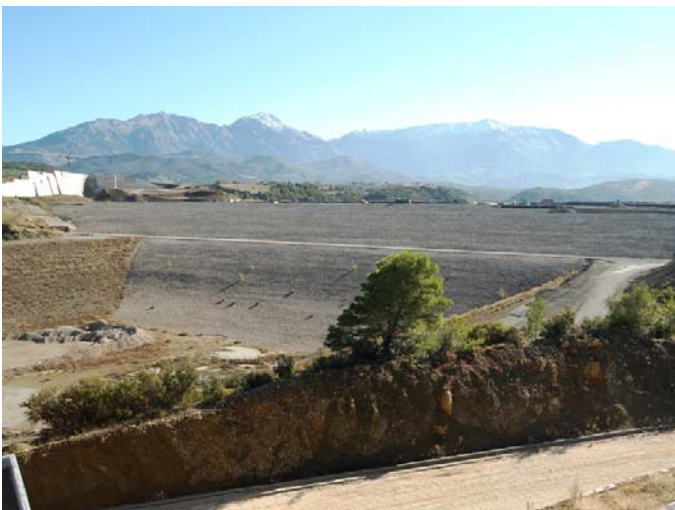
Patras Water Supply - Asterion Dam
