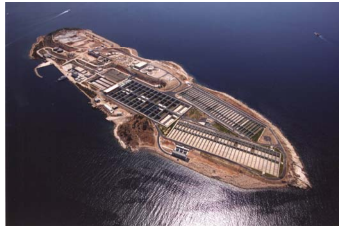
Athens Wastewater Biological Treatment Plant on Psyttalia Island
