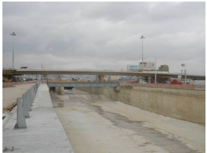
Kifissos River Flood Defence Works
