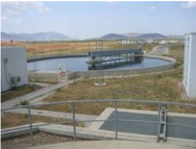
Wastewater treatment plant of New Athens International Airport
